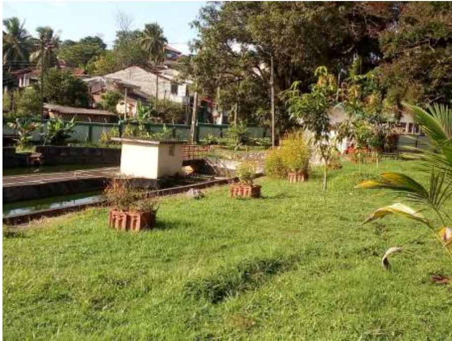
Existing sewerage plant
